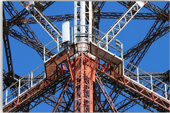
Small Cell on an electrical tower
