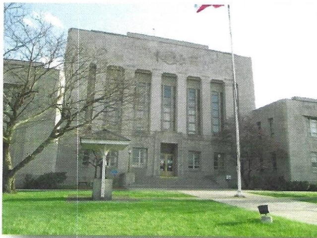
Mercer County Courthouse, Courthouse Road
