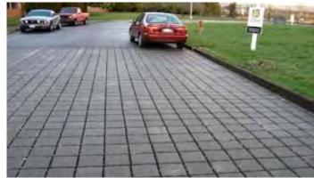
Figure 59: Permeable Pavement
