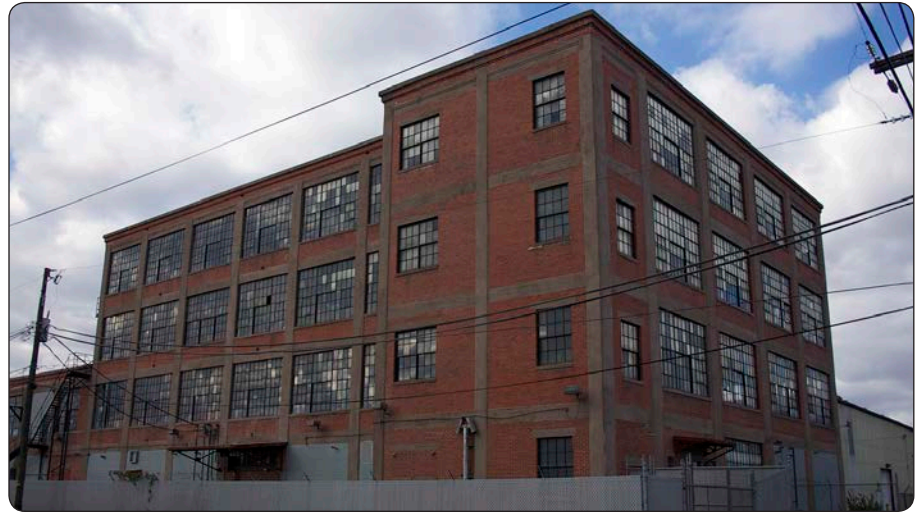
This former tobacco factory has two historically significant buildings, the redrying plant, which was built in 1910, and the factory, which was constructed in 1920.
