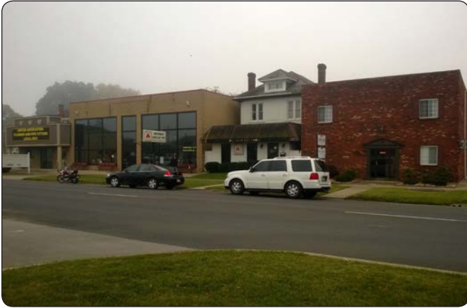
Several different development types exist in the downtown transition area.
