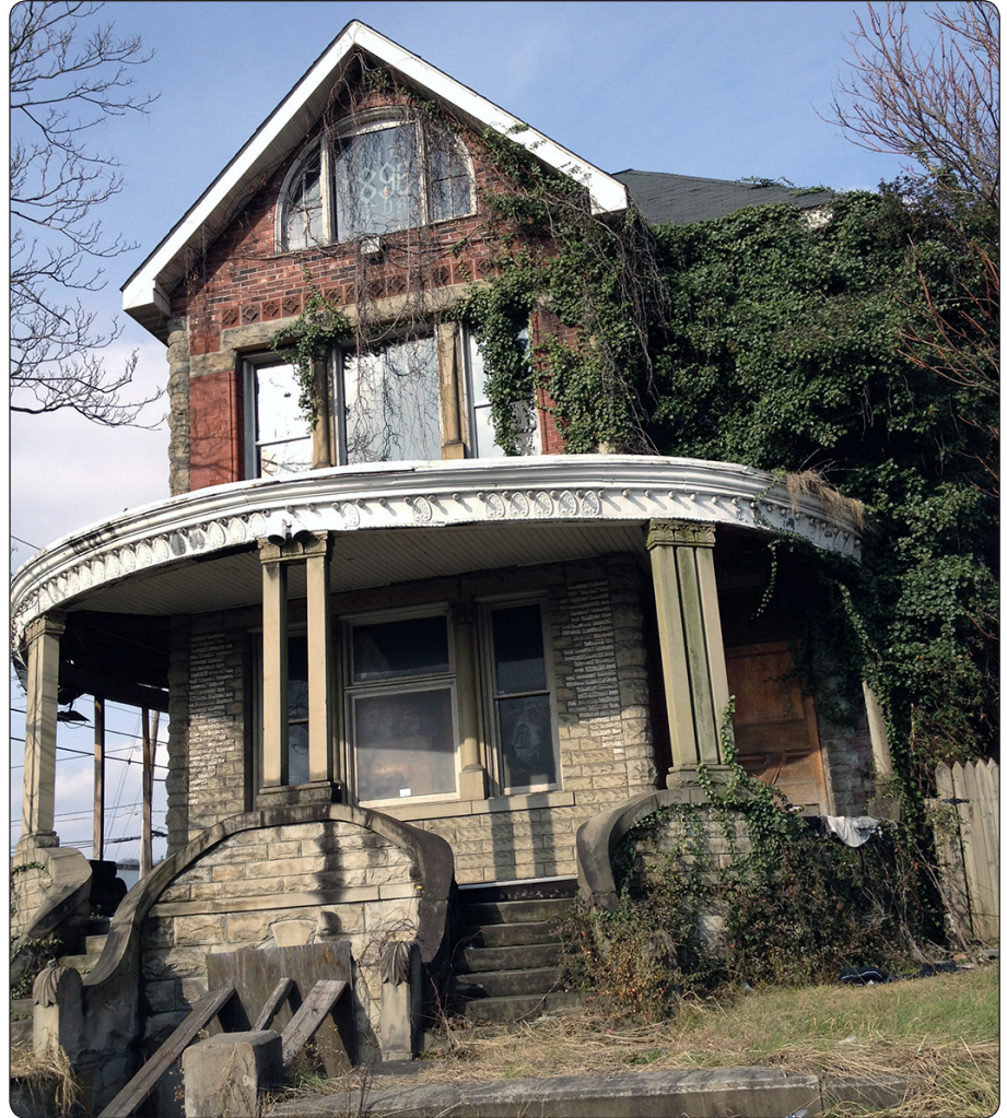
This former house and bar located on 3rd Avenue is a good example of historic housing that has fallen into disrepair after years of absenteeism.
