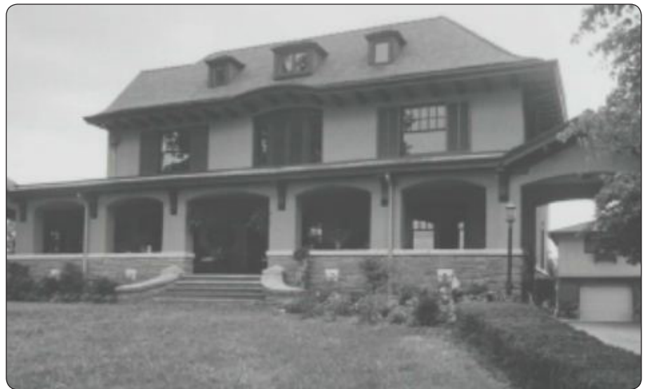
The Hawthorne Historic District is significant due to the Colonial Revival style of architecture and its association with several well-known Huntington architects and builders. Pictured above, the Staker/Angel House is the oldest known house on Hawthorne Way. It was built around 1900 for Mr. M.D. Angel who owned and operated Angel's Department Store located at 918 4th Avenue in downtown Huntington. (Photo from the WV State Historic Preservation Office)
