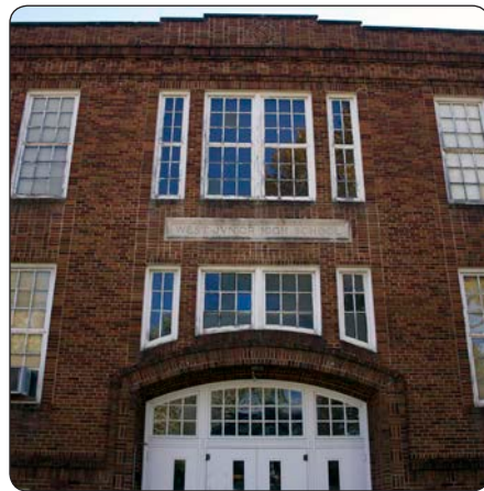
Positive reuse of West Middle School is important because it is no longer a neighborhood school.
