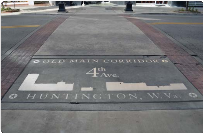
Pedestrian crossings are a part of the Old Main Corridor improvements.
