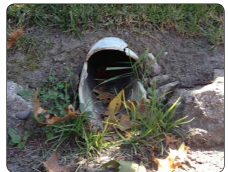
Disconnecting gutters from drains may help reduce flooding issues.
