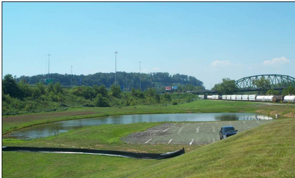
Picture 26 – The pond at Fort Neal Park was built to help mitigate stormwater runoff from the Elite Sports Center and new skate park. The retention pond will also serve as a recreational amenity, complete with walking path, shade trees and benches.
