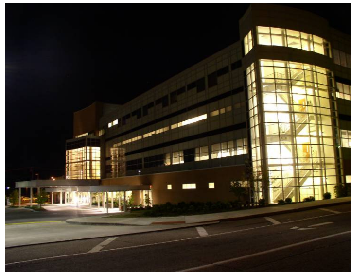
Picture 2 – The new addition at Camden Clark Hospital
