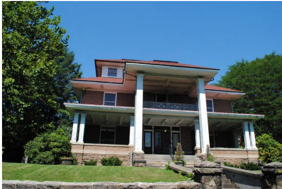
Historical Preservation (Front Ave)
